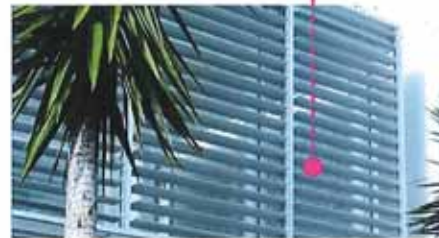
HORIZONTAL SCREENING IN ALUMINIUM HS
